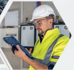
HVAC Control System Technician
